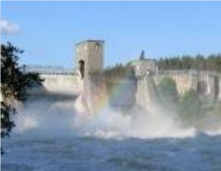
Imatra hydroelectric plant
